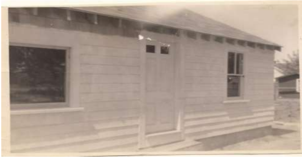
The home as it appeared when finished in 1950's Edgar and Loretta lived here until their death.
